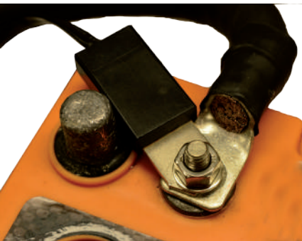
Fig 2.5(b) Temperature Sensor Installation
