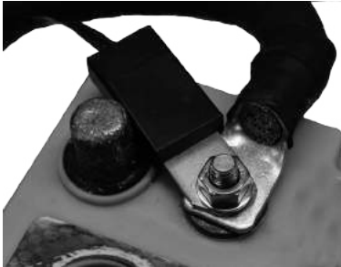
Fig 2.5(b) Temperature Sensor Installation
